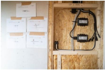
The more work steps are already carried out in the production halls, the easier the work becomes for the fitters on the construction site - this also applies to the electrical installation. This is where WOLF relies on the prefabricated, pluggable PREFAB solutions from Wieland Electric. (Image: Wieland Electric)
