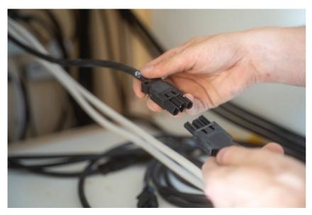
Plug-in electrical installation solutions, such as those that Wieland Electric has been offering for decades in the building sector, also enable rapid installation in modular construction and contribute to greater planning reliability. (Image: Wieland Electric)
