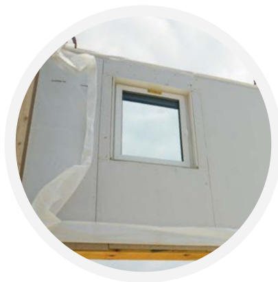
Prefabricated house construction, modular buildings
