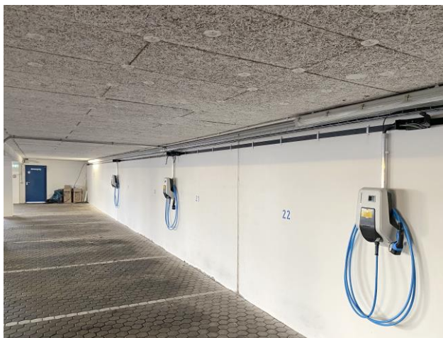
Figure 4: podis® energy bus system as used by Wieland Electric/@PaechElektro
