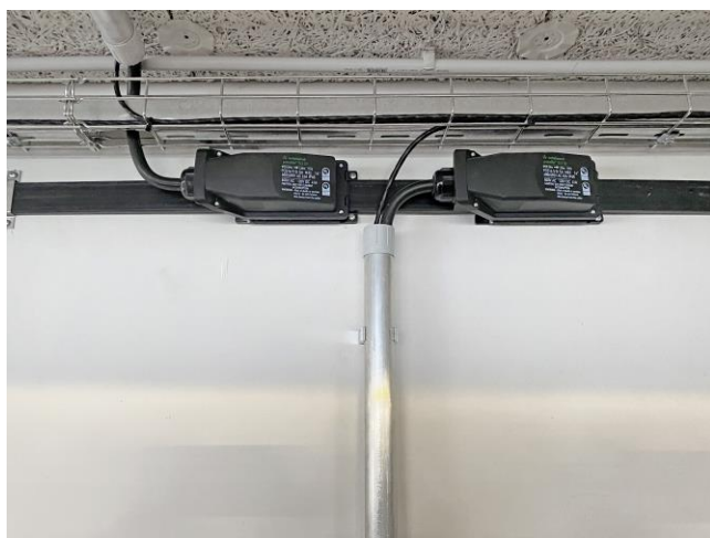
Figure 6: podis® energy bus system from Wieland Electric/@PaechElektro
