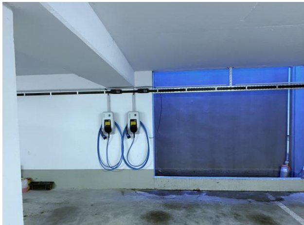
Figure 2: podis® energy bus system from Wieland Electric with boxes/@PaechElektro
