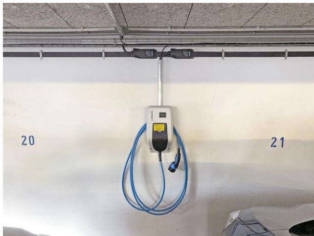
Figure 5: podis® energy bus system from Wieland Electric with box/@PaechElektro
