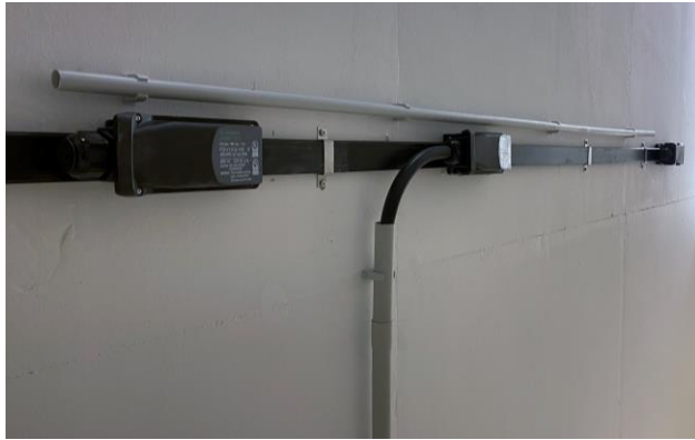
Figure 3: podis® energy bus system from Wieland Electric/@PaechElektro
