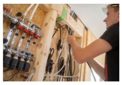
Wieland PREFAB also scores highly in buildings and building components that are serially produced using drywall construction and, thanks to its plug & play functionality and high degree of prefabrication, enables simple, fast and safe installation of the electrical infrastructure. (Image: Wieland Electric)
