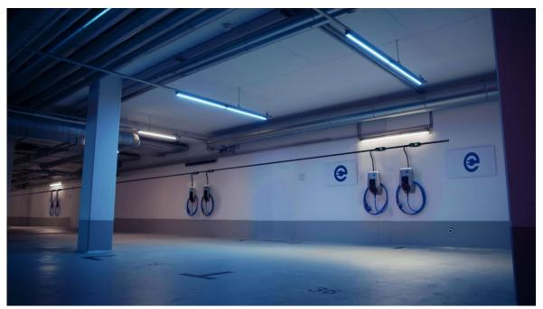
This is how decentralized energy distribution works. One flat cable can serve up to 20 charging stations.
