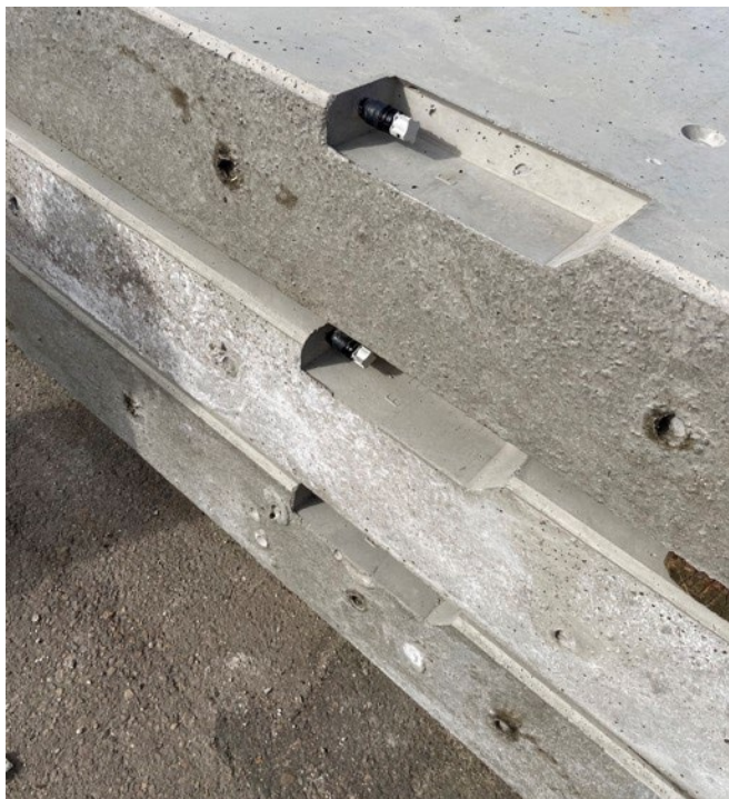
The RST® system from Wieland Electric enables installations to be cast into prefabricated floors and walls, making them "pluggable" on the construction site. (Image: Isolectra BV)
